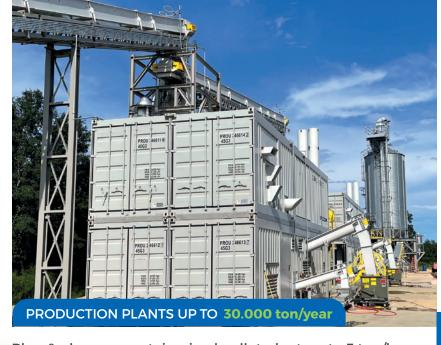
Plug & play: our containerized pellet plant up to 5 ton/h. PelletBox by Prodesa combines the reliability and quality of PRODESA pellet plants with the versatility of a containerized plant.
